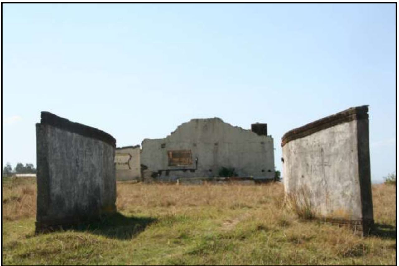
FIG.71: BUILDING AT LSS065
