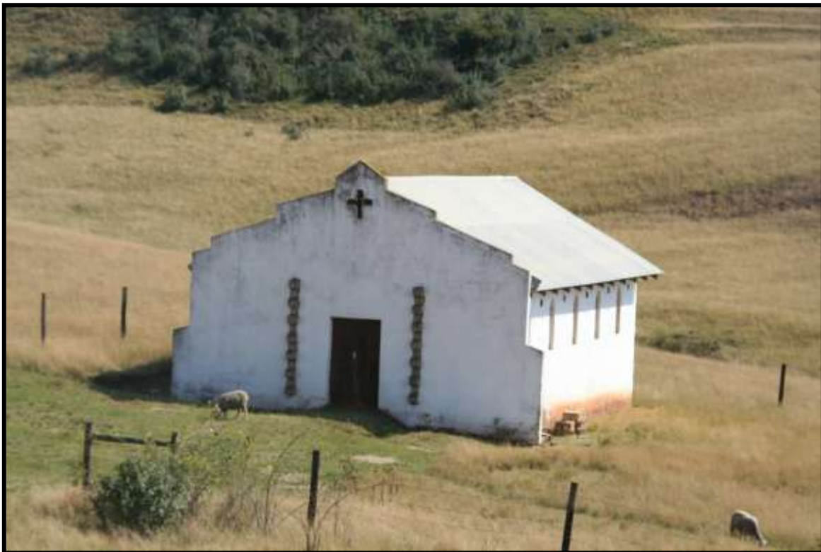
FIG. 39: CHURCH AT LSS039
